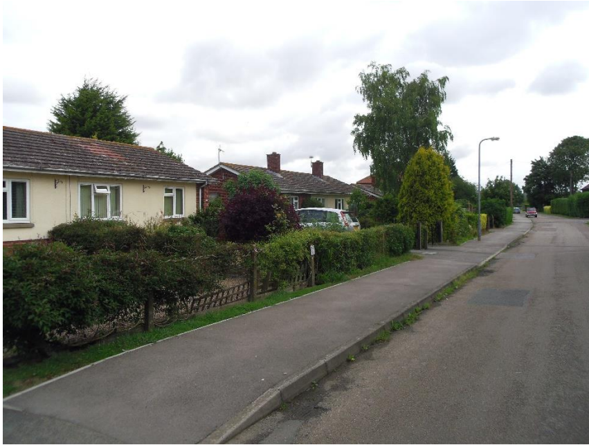
Figure 47 Back Lane Bungalows
