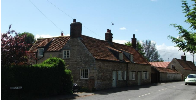
Figure 35: Lincoln Road is host to a row of fine vernacular properties
